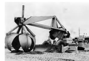
LeTourneau prototype excavating machine fitted with orange peel type positive-pressure grab bucket operated by geared racks, Longview plant, 1964
